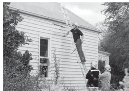
Carisbrook firefighters check the building after the fire was extinguished.
